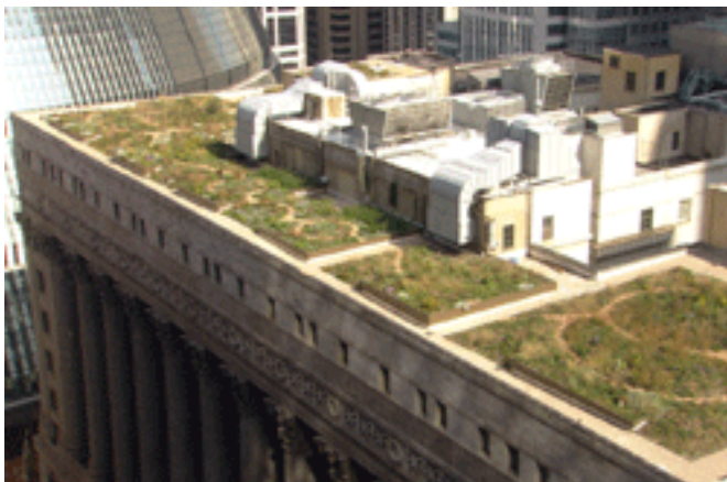
Figure 2: Green Roof atop Chicago’s city hall
